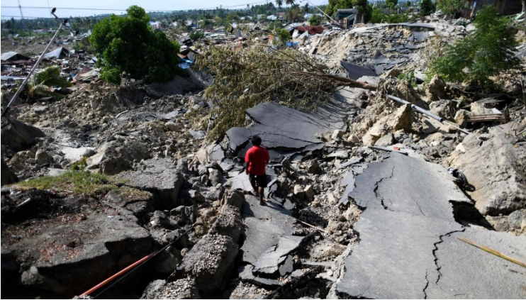
Figure 1.34: Liquefaction, Indonesia 2018.
