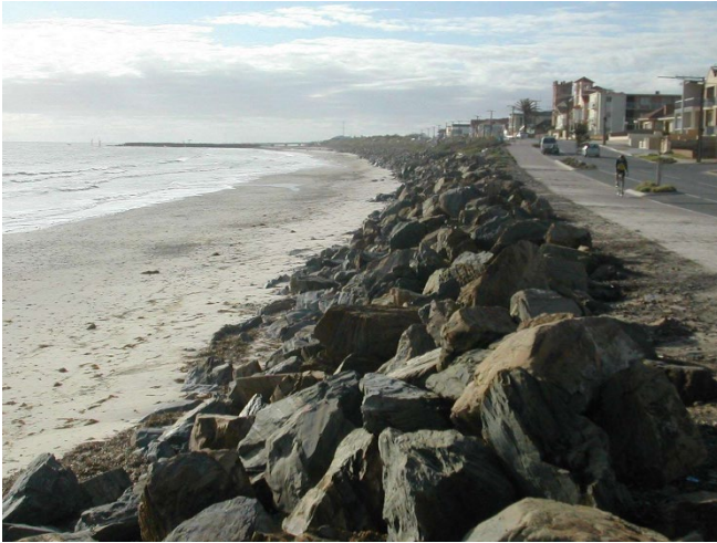
Sea walls protecting beach front homes from coastal erosion. Pictures from the North Coast of NSW where a road has been undermined by coastal erosion and an erected sea wall along Adelaide's Sothern coastline to protect homes.
