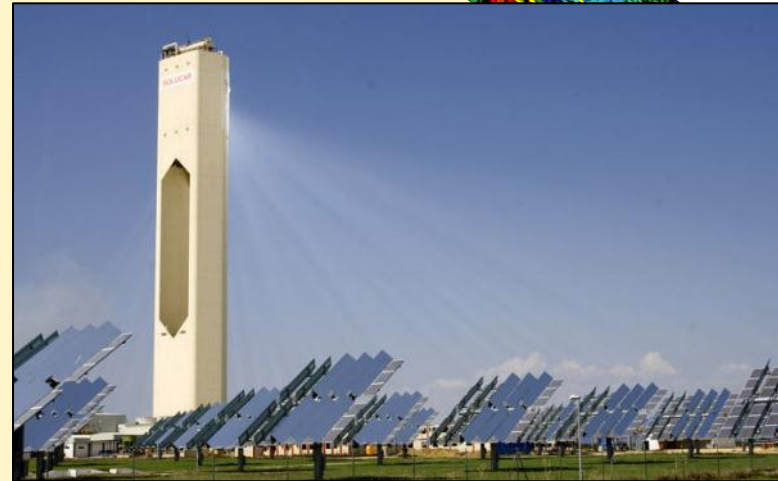
Solar thermal power plant
