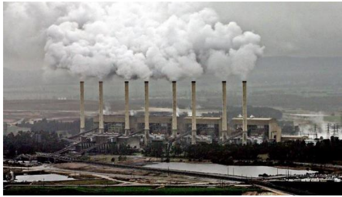
Hazelwood power station (Victoria) in full operation when it could produce ~25% of Victoria's electricity requirements from burning brown coal (lignite) ( http://reneweconomy.com.au/engie-flags-potential-closure-of-hazelwood-worlds-most-polluting-power-plant-26484/ )
