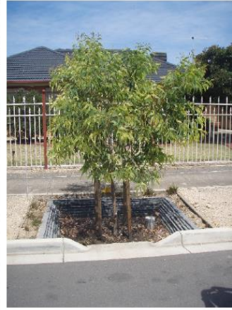
Tree pit bio-filtration system, Beechway Ave, Brooklyn Park
