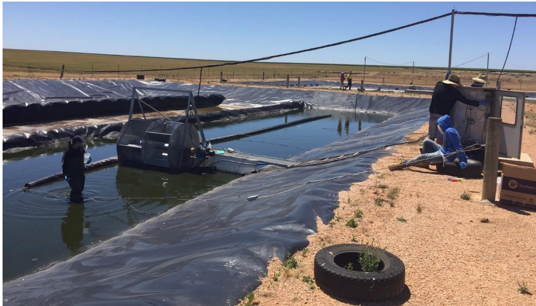
Flinders University researchers taking measurements from a High Rate Algal Pond (HRAP) at Kingston on Murray in the Riverland region of South Australia. HRAPs use algae to treat wastewater. Microalgae, produced as a by-product of the treatment process, can be utilised for biofuel production, as well as for animal feed and compost.
