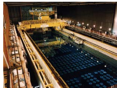
Fig. 6 a nuclear waste storage tank
